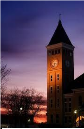
Saline County Courthouse
